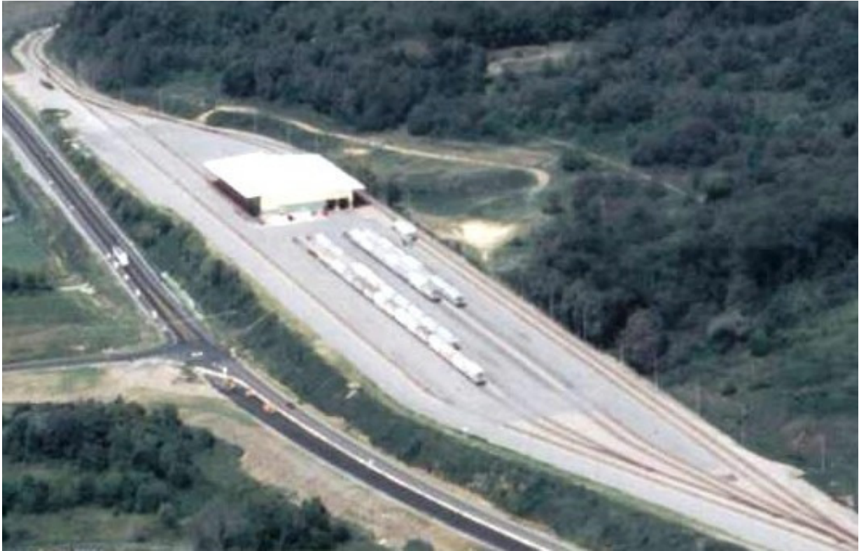
Aerial view of our Ethanol Rail-to-Truck Transloading Terminal in Mt Pleasant, PA
